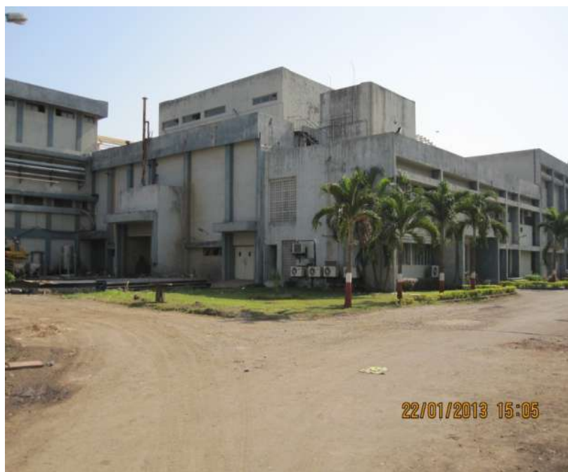
Fig. 3: Power Reactor Thorium Reprocessing Facility, (PRTRF), Trombay
