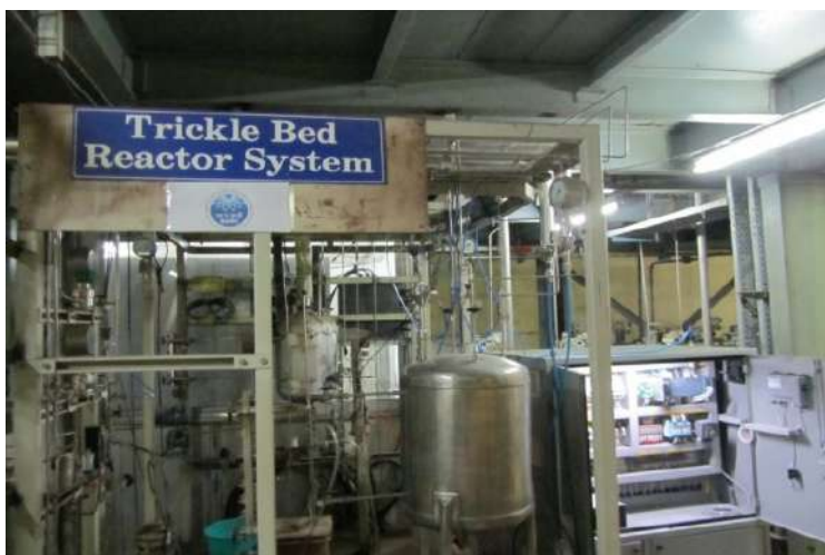
Figure 16: Test facility for LPCE and VPCE experiments
